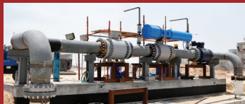
Mechanical work (Power / Oil & Gas Sector)
