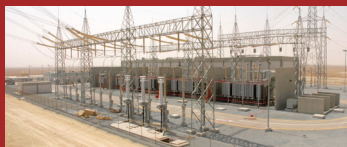
Electrical Work (Power / Industrial & Housing Project)
