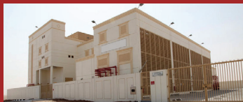
Civil & General Construction Work (Power / Oil & Gas Sector )
