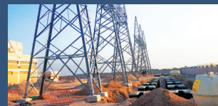
In Plant Civil
